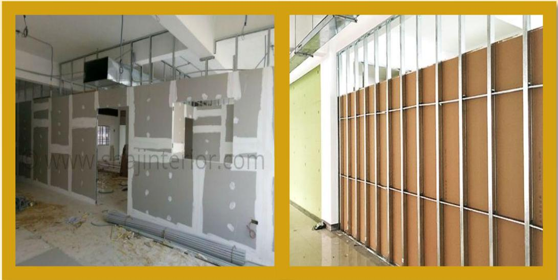
Dry wall partition system is widely used in offices and residential buildings for its easiness of installation. Dry wall partition system is made of durable galvanized steel. Usually it uses gypsum boards as surface material. Compared with bulky brick wall, it can greatly reduce the weight of building.
