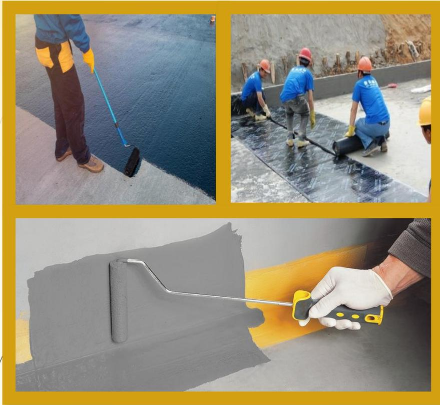
Waterproofing is one of the most important applications in a construction. Waterproofing improves the durability of many different surfaces in construction. Waterproofing is the formation of an impervious barrier over surfaces of foundations, roofs, walls, and other structural members. The function of the impermeable barrier is to prevent water penetrations. The building surfaces are made water-resistant and sometimes waterproof.
