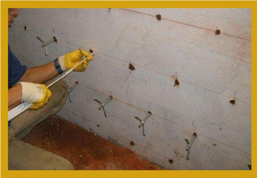
Water ingress can escalate project costs and lead to many other problems. The use of injection systems based on dual and single component polyurethane and acrylate resins are cost-effective and provide a high success rate.
