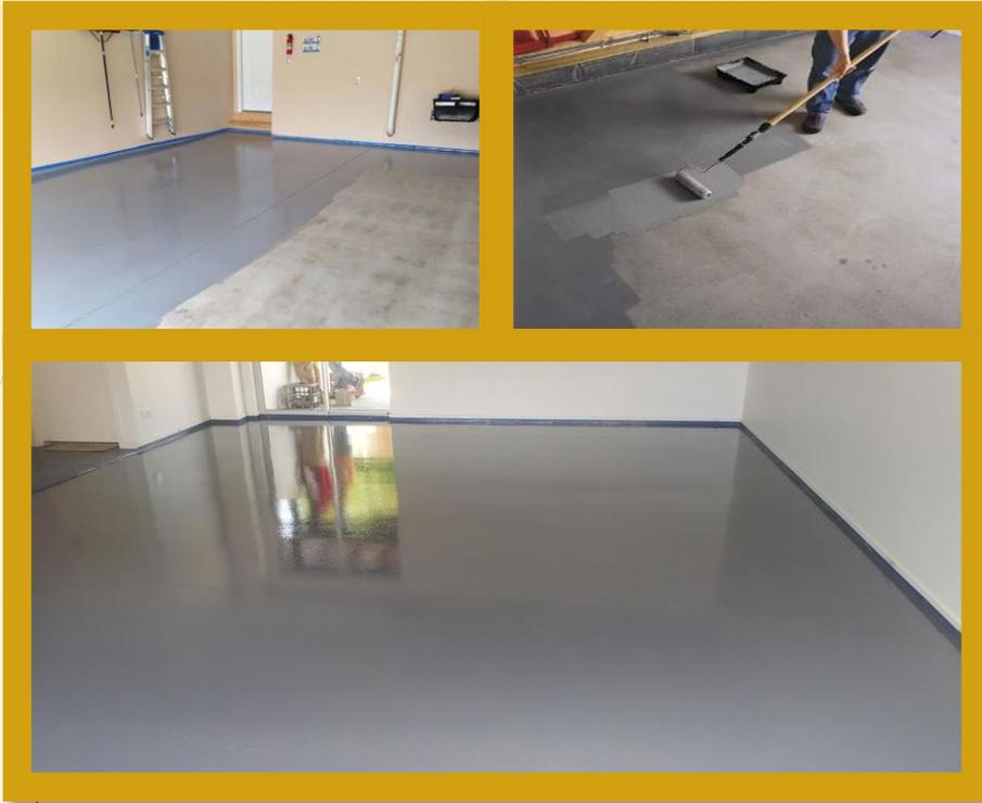
Epoxy floor coatings are commonly used for commercial and industrial flooring. Epoxy coatings are normally applied over concrete floors to provide a high-performance, smooth, and durable surface that can last many years and withstand heavy loads. Many industrial sites, warehouses, and commercial buildings rely on epoxy floors to maintain clean and safe conditions for workers, equipment, and inventory.
